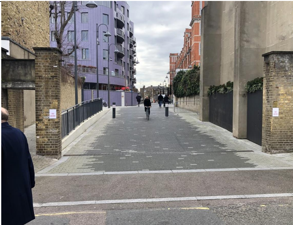
Figure 7: Main site exit at Almeida Street
